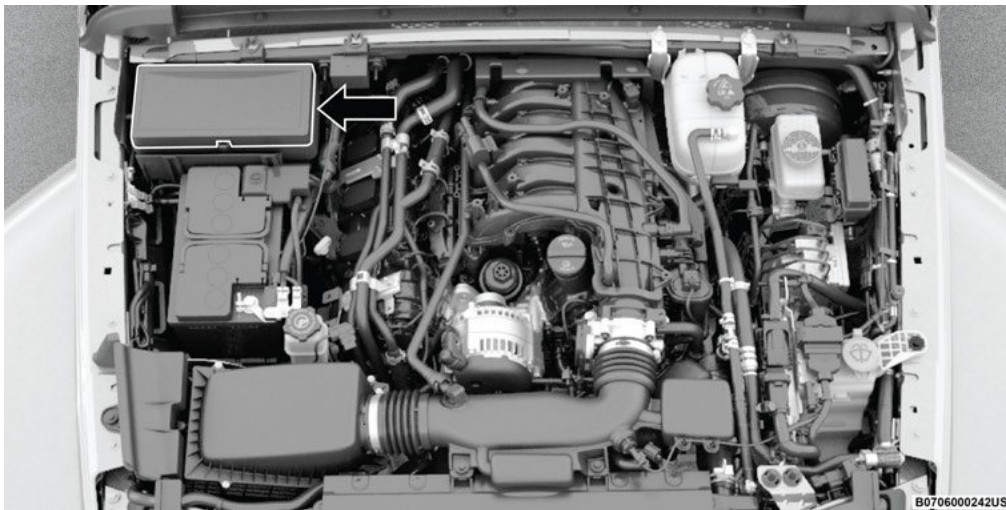
Power Distribution Center Location - Gasoline Engine
