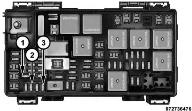
Power Outlet Fuse Locations
